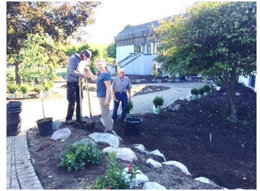
Norm Jolin, Sr. supervises the installation of plants and ground cover.
