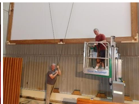
Thom and Jim install the decorative outer frame.
