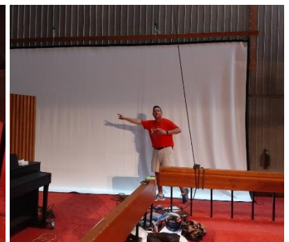
The screen material is laced to the frame and raised to be attached to the wall.
