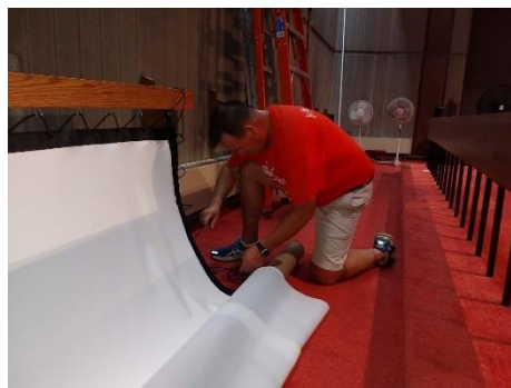
The screen material is laced to the frame and raised to be attached to the wall.
